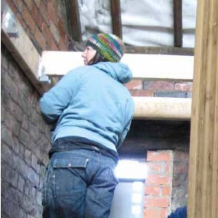
House renovations in Leeds.
